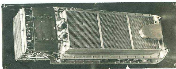
**Figure 6.** Soft X-ray payload flown on RH 560 rocket.
