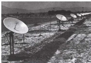
**Figure 4.** Kalyan Radio Telescope (1965-1068) consisting of 32 dishes of 5.6 ft. diameter each (24 in 2000 ft. East-West array and 8 in 800 ft. North- South array).
