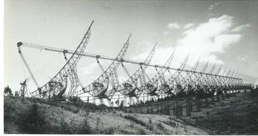
**Figure 5.** Ooty Radio Telescope consists of a 500m long and 30m wide parabolic cylindrical reflector. Its long axis of rotation is parallel to the axis of rotation of the Earth. There are 1054 dipoles receiving radiation at a frequency of 325 MHz (Swarup et al. 1971).
