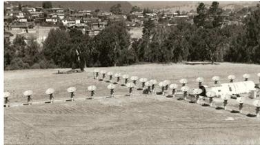
**Figure 2.** Stanford Heliograph consisting of 32 parabolic dishes of 10ft diameter each for daily mapping of solar radio brightness distribution at 3100 MHz (Bracewell and Swarup 1961)
