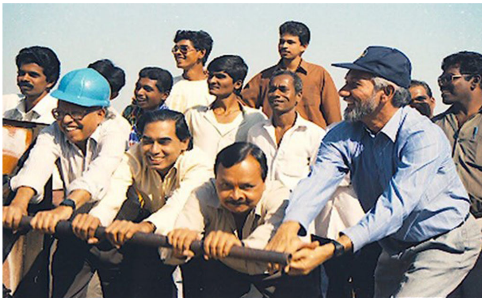
Figure 6. The 45 m diameter antennas of the GMRT were constructed at ground level and then raised onto their altitude–azimuth mounts by hand-operated winches. Here Govind (front row, light-blue hat) lends a hand to the winching operation. Others in the front row (from left to right) are S. C. Tapde (the GMRT project engineer), B. S. Mathikere (the engineer at the GMRT site) and Vijay Kapahi (who succeeded Govind as centre director, NCRA). Used with permission of TIFR.
