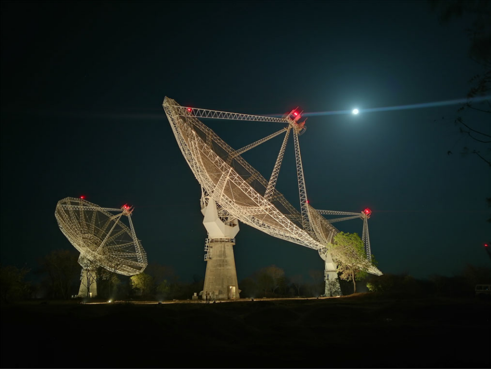
Figure 7. Three of the 30 GMRT dishes. Each dish is 45 m in diameter, and the entire array is spread over a region about 25 km across. The signal from each antenna is brought to a central location via optical fibre for further digital processing. The GMRT is a national facility, but is operated under an ‘open sky’ policy. Astronomers from across the world can propose use of the GMRT; time is allocated purely on scientific merit as judged by an independent time allocation committee. The telescope is extremely versatile. Science done with the GMRT ranges from studies of the heliosphere to the very early stages of the Universe (the so-called Epoch of Reionization) and a whole host of phenomena at distances intermediate between these two. Photograph courtesy of National Centre for Radio Astrophysics, India.
